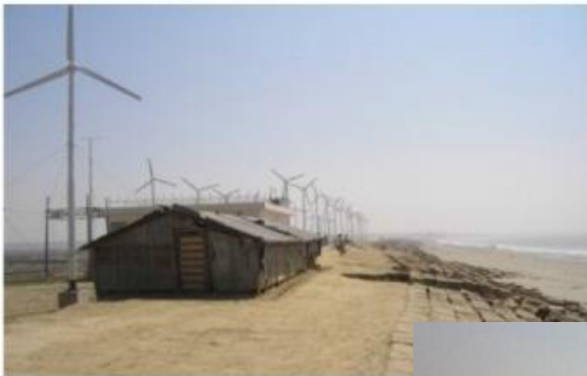
1000 kW Wind Battery Hybrid on Kutubdia Image source: BPDB, Implemented projects
